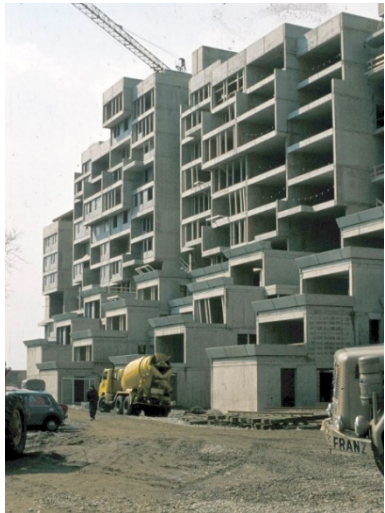
Fig. 8: Photo of the construction site after completion of the primary structure, © Walter Kuschel
